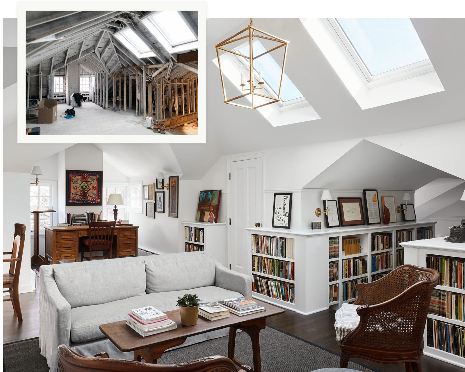
A PURE member's home during and after renovations following a home fire.
