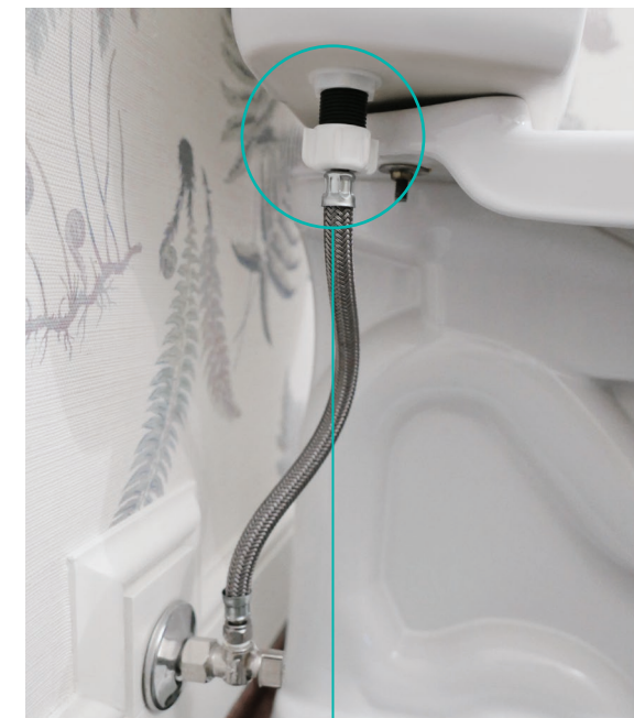
Plastic connectors attaching the toilet supply line can crack over time and cause significant water damage.
